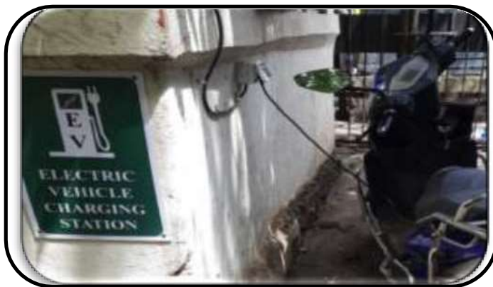
Electric Vehicle Charging Station
